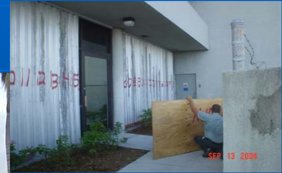
Installation of Hurricane Shutters prior to storm
