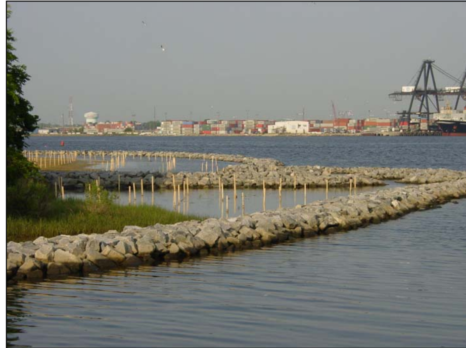
Wetlands Planting (Wetlands Restoration Area) North Side of Plum Point May 2004
