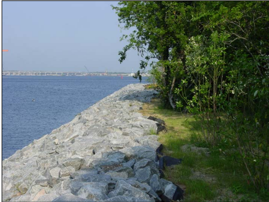
Rip Rap Shoreline Protection (River Clean-Up Area) South Side of Plum Point May 2004
