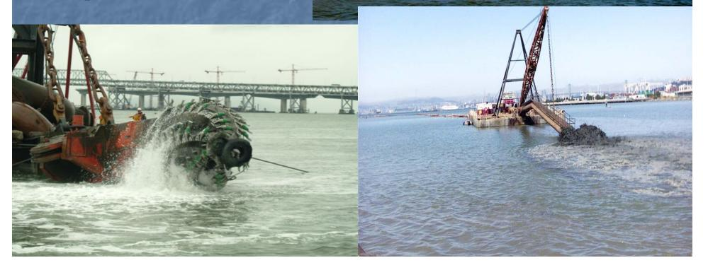
Hamilton Wetlands Disposal •2.6 million CY 14 nautical miles away, will P require hydraulic offloader and **Boosters**  35,000 feet pipelines to install and pump through Tight Fill Requirements (+/- 0.25) ft) Directly Adjacent to High Dollar **Residential Areas**
